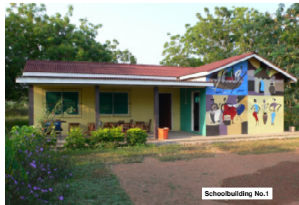
School Building No.1
