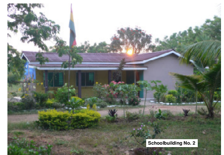
School Building No.2
