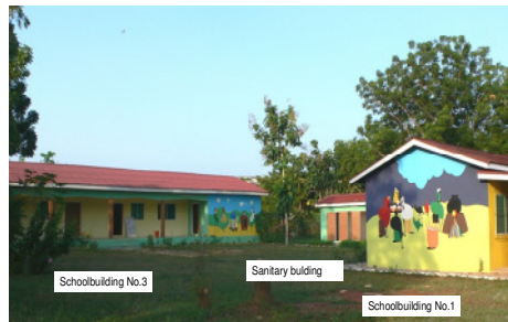
School Building No.3, Sanitary Building,
